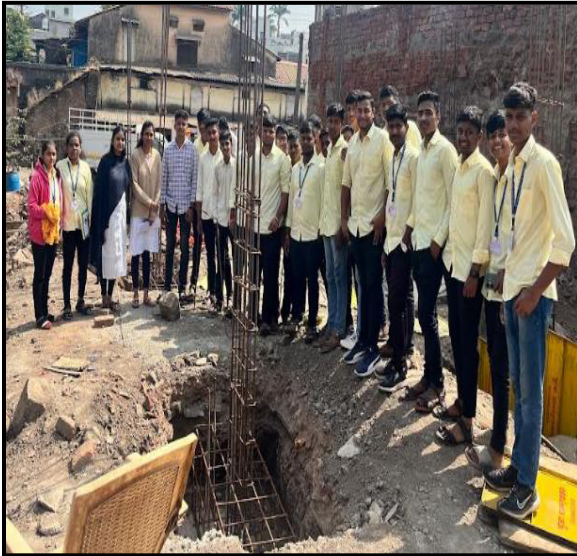
Residential Building Visit Place : Kodoli Date :31/01/2024.
